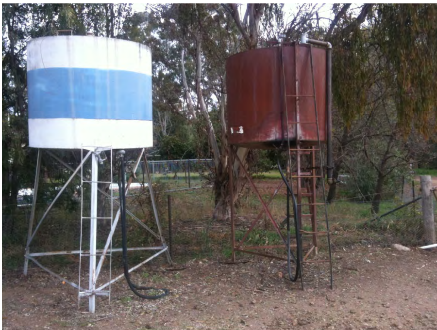
Photo 11 – Diesel storage tank on the left and unleaded storage tank on the right
