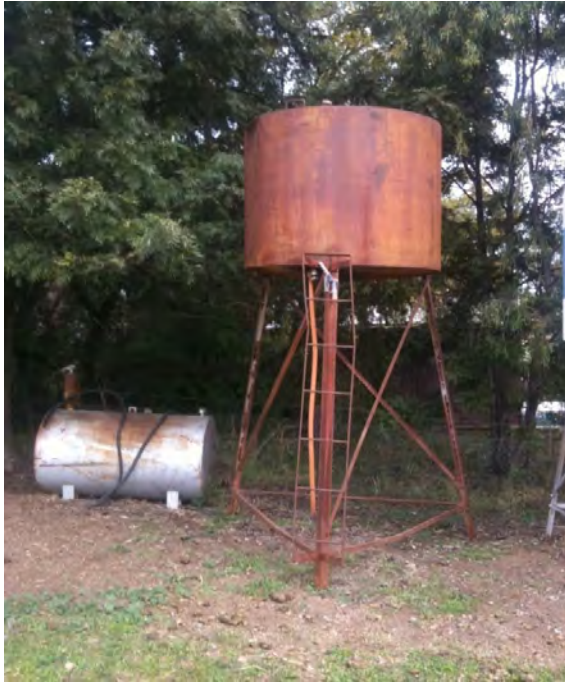
Photo 12 – Diesel storage tank and a portable storage tank
